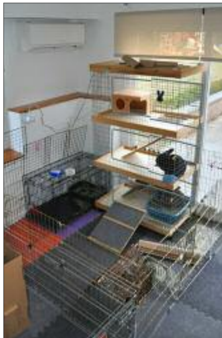
AC/heat unit mounted at the top.
